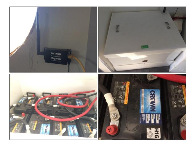
Finally there are the three battery storage boxes. Each box contains 8 batteries, for 24 batteries total. The batteries are labeled "Sealed Deep Cycle, Maintenance Free, AGM Battery". They are Crown 1 model number 6CRV390, 6 volts, 390 (20HR) A.H. Rating.
