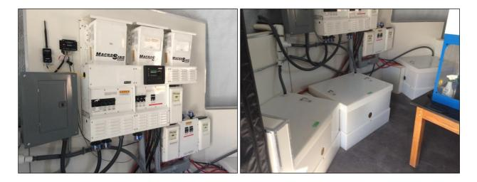
Inside the Science Dome, a good section of the wall on one side is taken up by electrical conditioning equipment and batteries which are stored in three large boxes on the floor.
