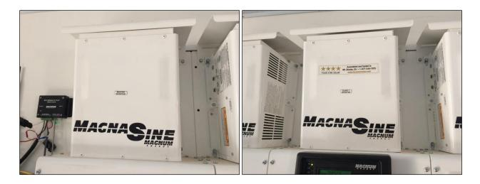
There are three white boxes labeled "MagnaSine Magnum Energy". The first is labeled "Master Inverter". The others are labeled "Slave 1 Inverter" and "Slave 2 Inverter". I am not sure of the precise configuration or why there is a Master, Slave 1 and Slave 2, but these are clearly the invertors that take DC put out by the solar panels and stored in the batteries and convert it to AC.
