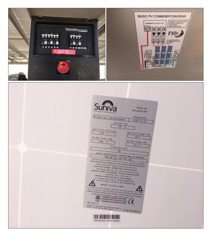
This is a sizeable solar array! There are a total of 45 individual panels. The solar cells on each panel measure ~37.5" x 75", or 3.125 ' x 6.25' = ~19.5 sq ft ea. The total area of solar cells is therefore ~878 sq ft. I captured a picture of the label on the underside of one of the panels. It indicates a maximum power production per panel of 335W. With 45 panels, this is a max power output from this array of 15,075 W (15kW).
