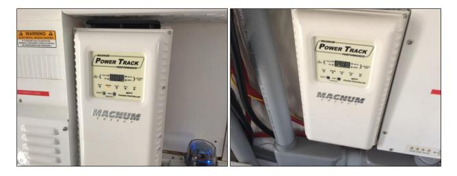
There were three white Magnum energy boxes labeled "Power Track Performance" and "MPPT Charge Controller". MPPT stands for "Maximum Power Point Tracker". These are DC to DC converters that match the output voltage of the PV array to the optimal voltage needed to charge the batteries.
