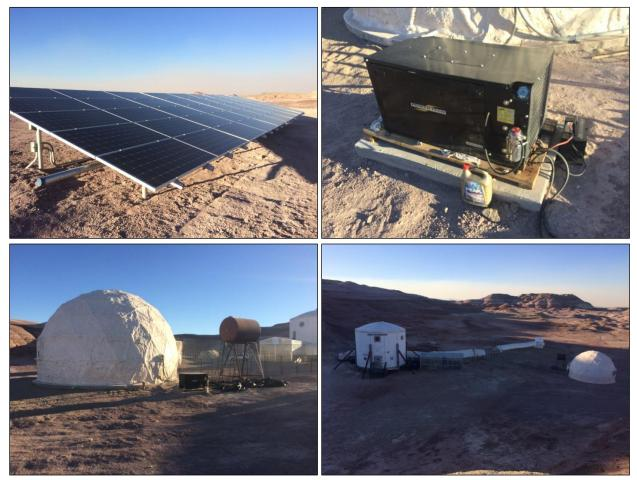
Also on site, and of particular interest to this engineer, is power systems infrastructure. This consists of a large solar array, a generator, and a fuel storage drum for the generator. More on this later.
