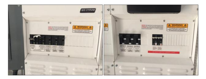
There were breakers that indicated they would be used for Inverter AC Bypass, Invertor AC Output, Inverter AC Input, Inverter DC Disconnect, C.C. #1 PV Array Input and C.C. #1 PV MPPT Output.
